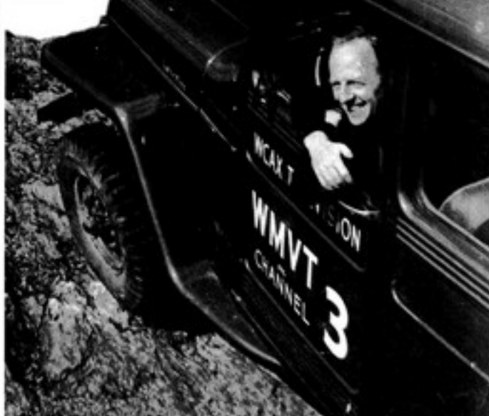
Stuart Martin "on the edge" looking down from the heights of Mount Mansfield during the construction of WCAX in 1954. Word has it that this is his favorite photo of those days.
